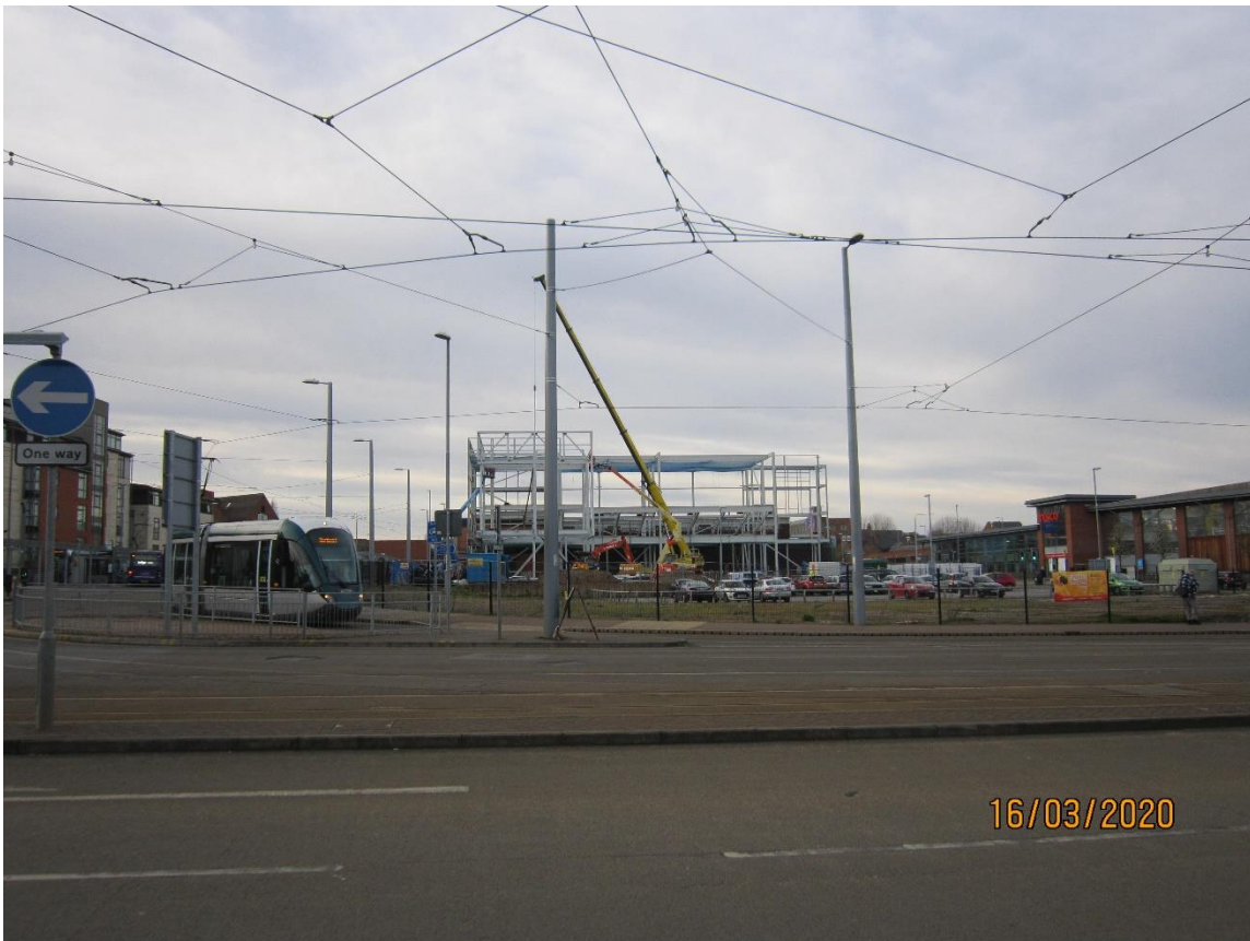
Site viewed from Middle Street with cinema building under construction
